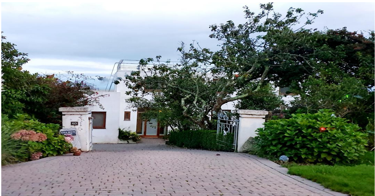
Fig 3: Gull Rock House – a listed art deco style house
